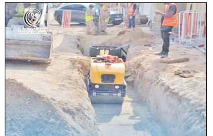
Maintenance work ongoing in Qurtoba.
