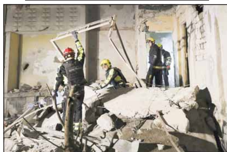
Emergency services workers move rubble after a Russian strike on a residential building in Kharkiv, Ukraine on Sept 22. Russian strikes hit high-rise apartment blocks in Ukraine's city of Kharkiv, leaving dozens wounded in a second consecutive nighttime attack this past week. (AP)
