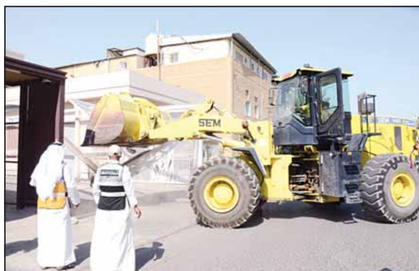
Kuwait Municipality officials conduct demolition of one of the encroachments.
