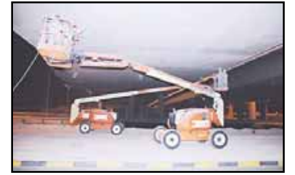
Photo by Rizk Taufiq Painting a bridge.
