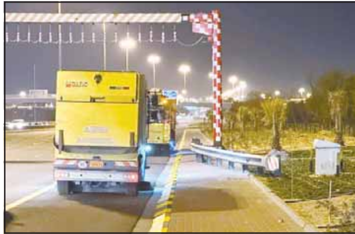
Municipality trucks ready to carry out the works.
