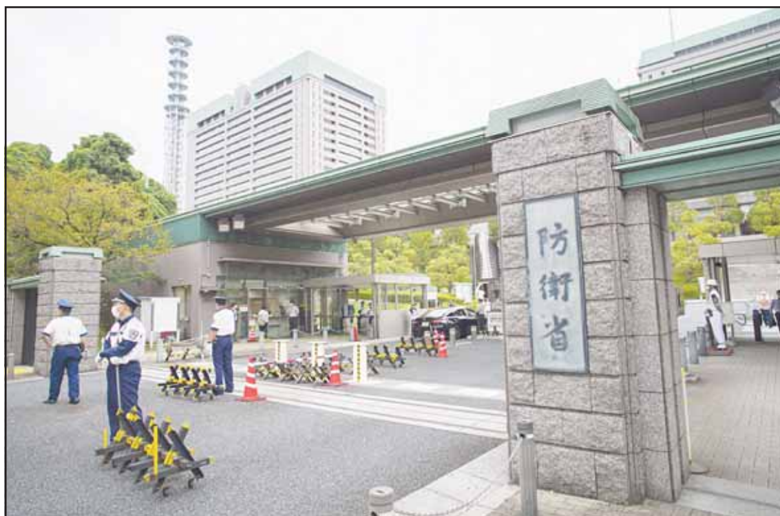
This photo shows an exterior view of the Defense Ministry of Japan with its sign at the main entrance in Tokyo on Sept. 17, 2021. (AP)
