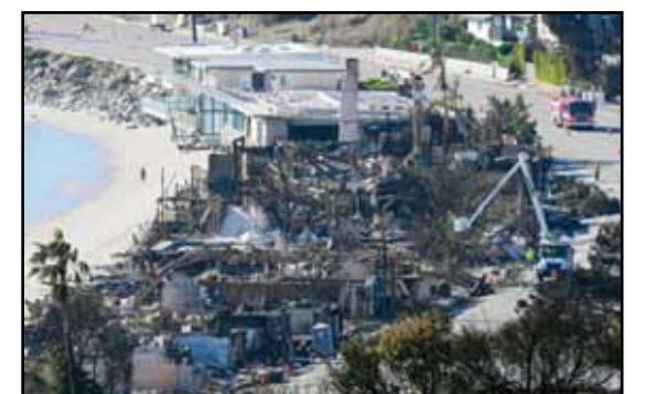
Homes along Pacific Coast Highway are seen burned and damaged while a few still stand after the Palisades Fire, Jan. 12, 2025, in Malibu, Calif. (AP)
