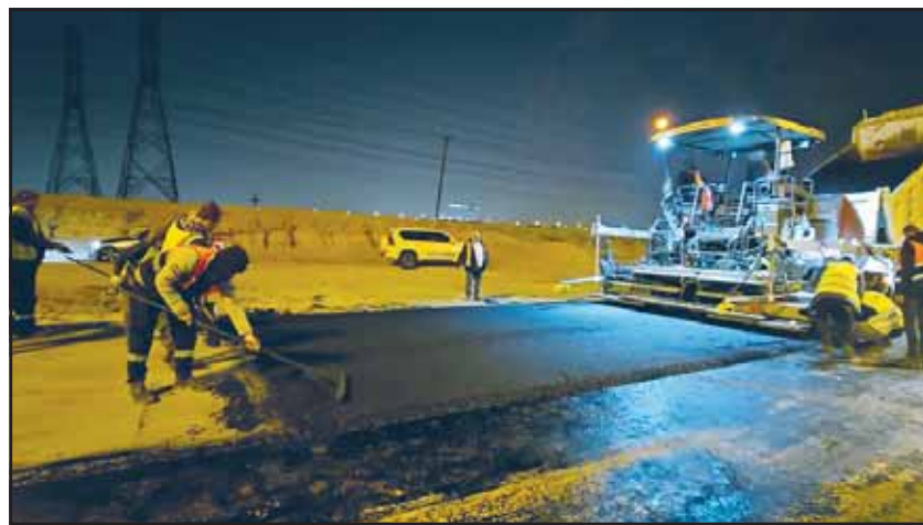
Road repairs underway in a residential area.
