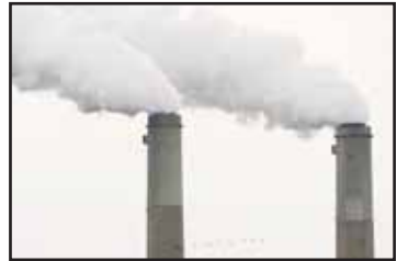
The Jeffrey Energy Center coal-fired power plant operates near Emmett, Kan., Jan. 25, 2025. (AP)
