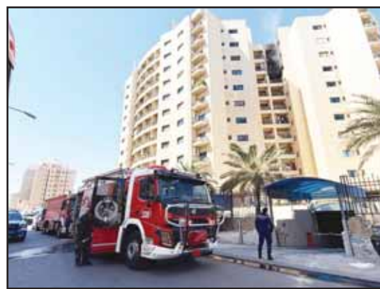
Traces of fire seen on the building.
