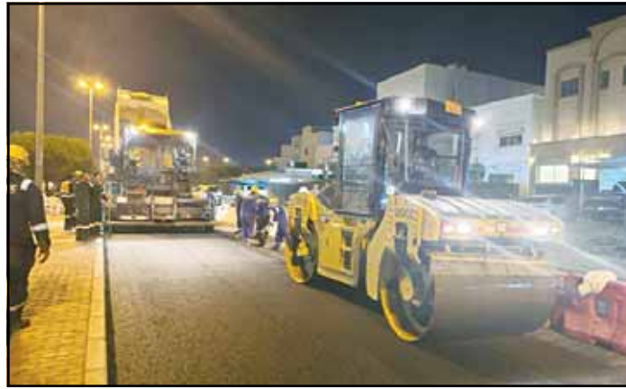
Road maintenance underway in Jaber Al-Ali.
