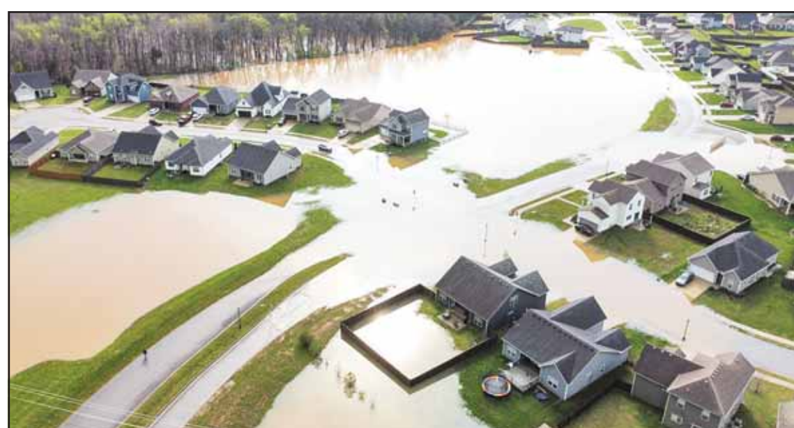
Flood waters cover the entryway to the Weather Stone subdivision off Russellville Road in Bowling Green, Kentucky on April 4 after excessive rainfall Thursday into Friday drenched southcentral Kentucky with more than four and a half inches of rain. (AP)
