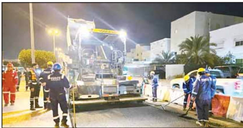
Road maintenance underway.
