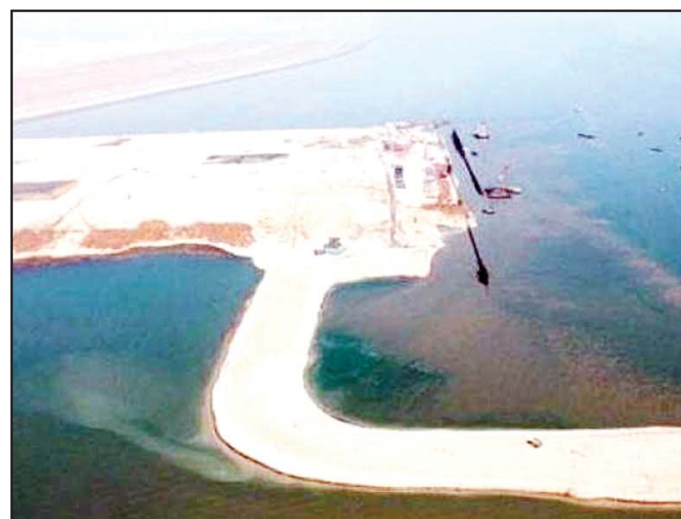
Aerial shot of Mubarak Port project.
