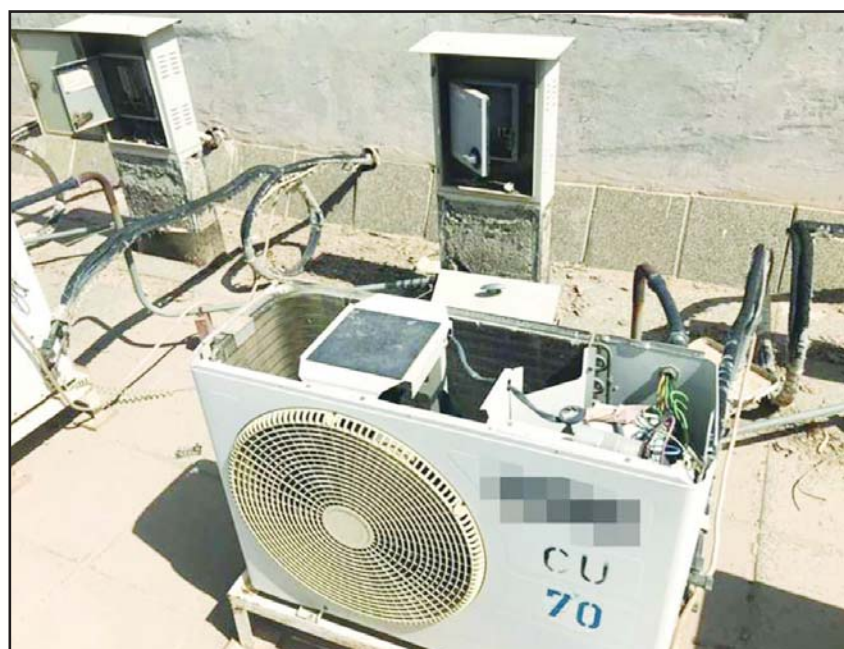
AC units are repaired at one of the schools.
