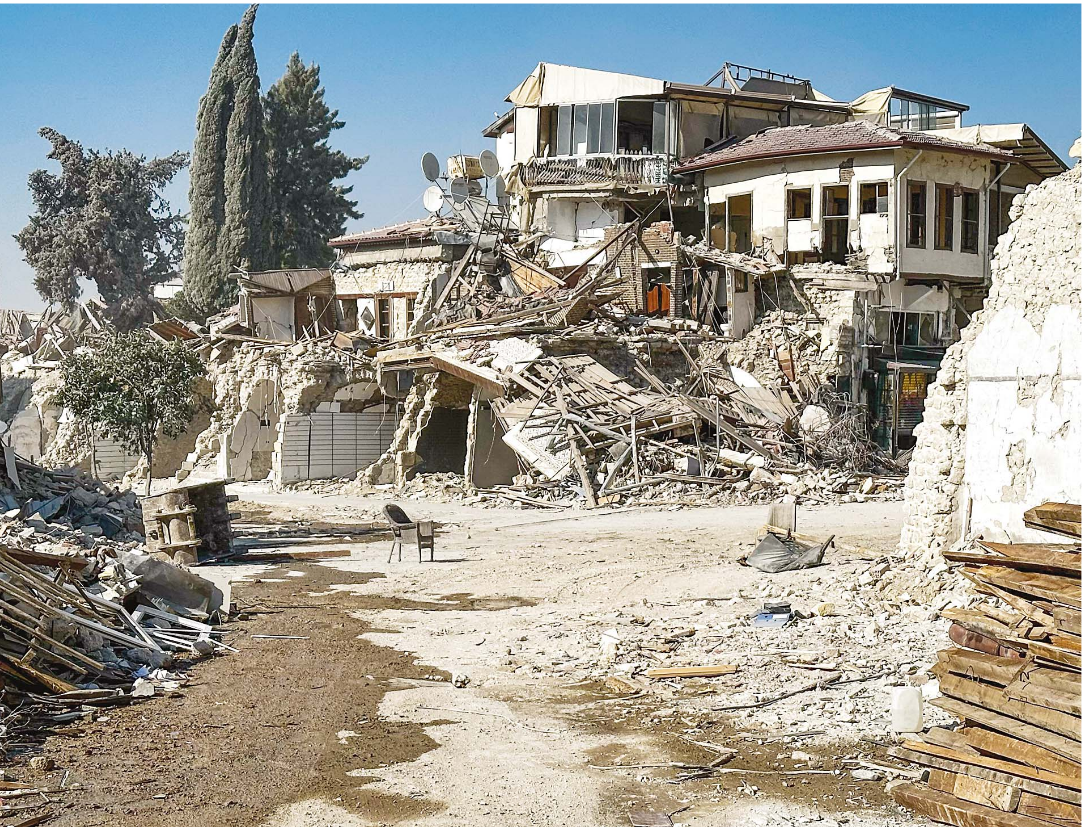
The remains of buildings destroyed during the earthquake are pictured in Antakya, southeastern Turkey and 10 other provinces in southern Turkey on the morning of February 6th. Over 50,000 people died, and Saturday, Aug. 5, 2023. Six months ago, a devastating 7.8-magnitude earthquake hit the Kahramanmaraş hundreds of thousands were left homeless, sheltering in tents and other temporary accommodation. (AP)
