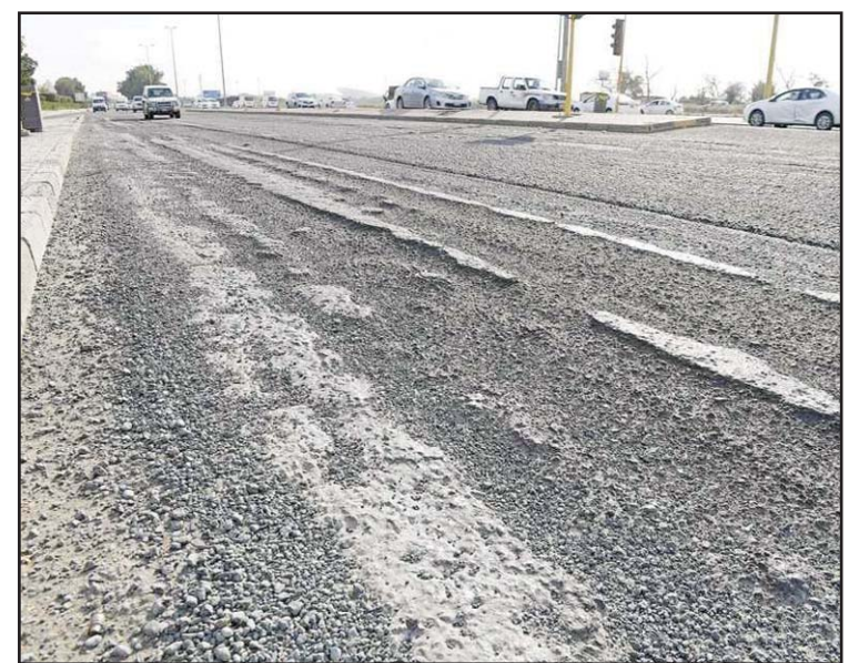
Ministry of Public Works plans to maintain and radically rehabilitate roads.
