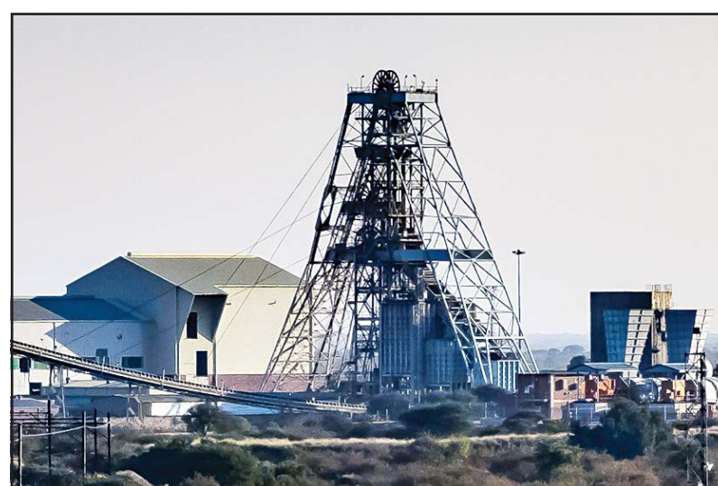
This is an undated photograph of Impala Platinum mine shaft 11, provided by Implats on Nov 28, near Rustenburg, South Africa. An elevator suddenly dropped around 200 meters (656 feet) while carrying workers to the surface in a platinum mine in South Africa, killing 11 and injuring 75, the mine operator said Tuesday. It happened Monday evening at the end of the workers' shift at a mine in the northern city of Rustenburg. The injured workers were hospitalized. (AP)
