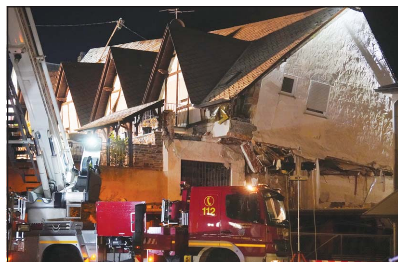
A fire department vehicle stands in front of a collapsed hotel in Kroev, Germany on Aug 7. Part of a hotel on the Mosel River in western Germany collapsed, leaving two people dead and several others trapped in the wreckage, authorities said on Wednesday. (AP)
