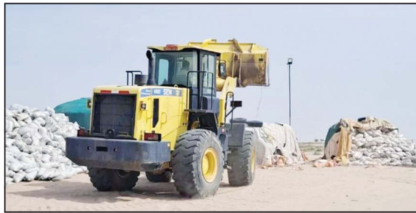
Encroachments being dismantled at 'Kilo 34' in Wafra. Al-Seyassah photo
