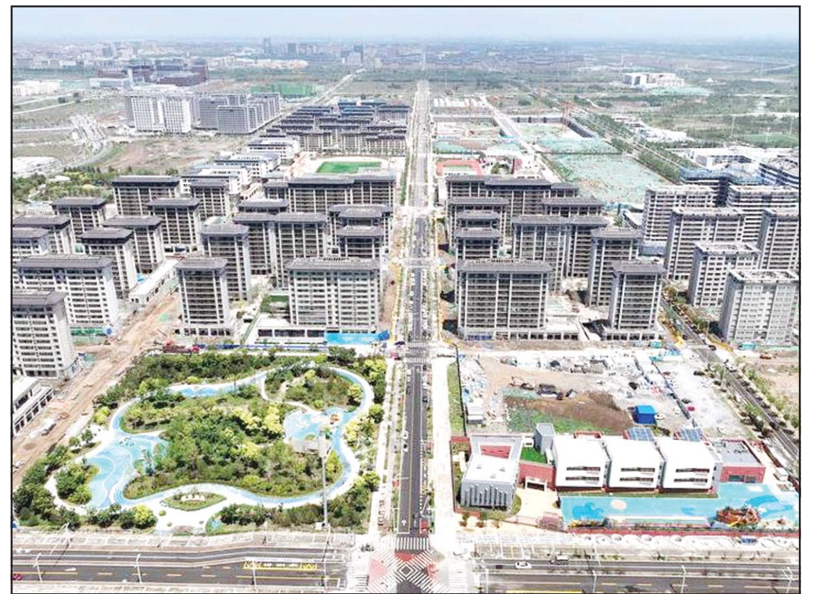
This aerial photo taken on July 4, 2023, shows the construction site of a residential housing project in the start-up area in Xiong'an New Area, north China's Hebei Province. China announced plans to establish the Xiong'an New Area on April 1, 2017, located about 100 km southwest of Beijing, aiming to build the area into a national model of high-quality development and a new engine for the modern economic system. The Political Bureau of the Communist Party of China (CPC) Central Committee held a meeting on June 30, 2023 to review the guidelines on a raft of policies and measures supporting the high-standard and high-quality construction of the Xiong'an New Area. The focus of the work involving Xiong'an has shifted to high-quality construction and high-level management, the meeting pointed out. XIONG'AN, July 7, 2023 (Xinhua)
