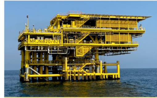
Oil Production Deck Module in Saudi waters
