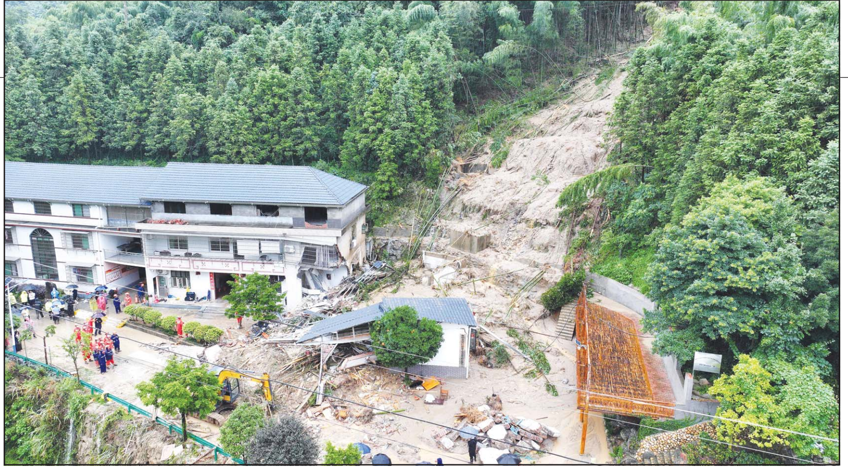
An aerial drone photo taken on July 28, 2024 shows the landslide site in Yuelin Village of Shouyue Town in Hengyang City, central China's Hunan Province. (Xinhua)
