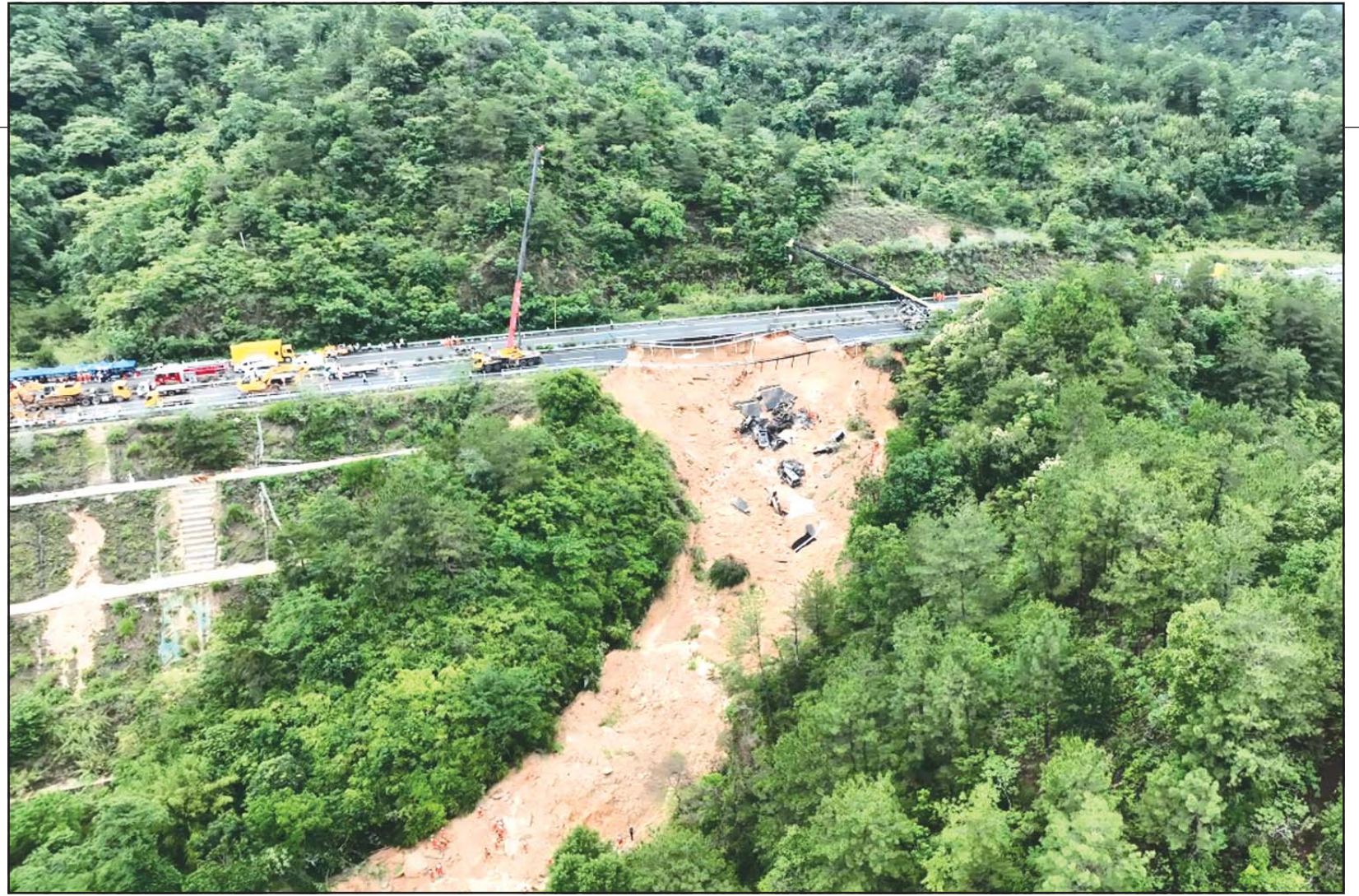
This photo taken on May 1, 2024 shows the site of an expressway collapse accident on the Meizhou-Dabu Expressway in Meizhou, south China's Guangdong Province. (Xinhua)
