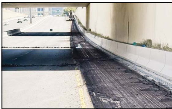
Work begins on tunnel road.
