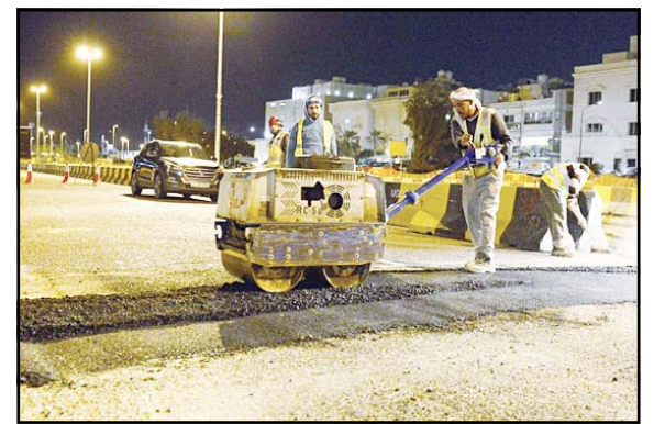
Patchwork continues on one of the roads.
