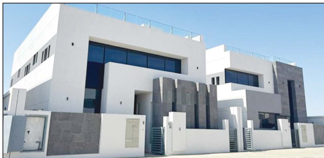
East Sabah Al-Ahmad housing project
